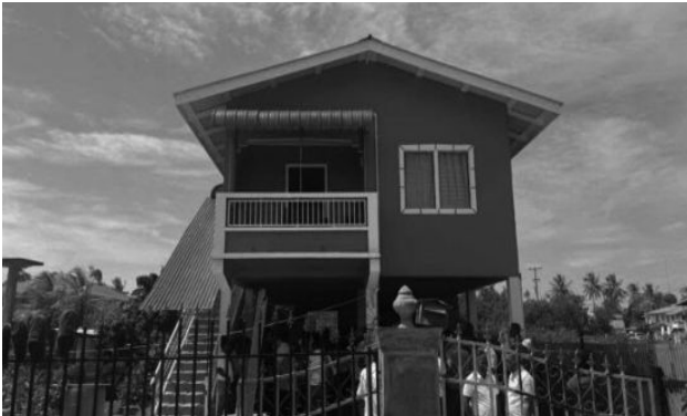
The newly constructed home of Jerry and Rosaline Alexander, who lost their home in a fire
