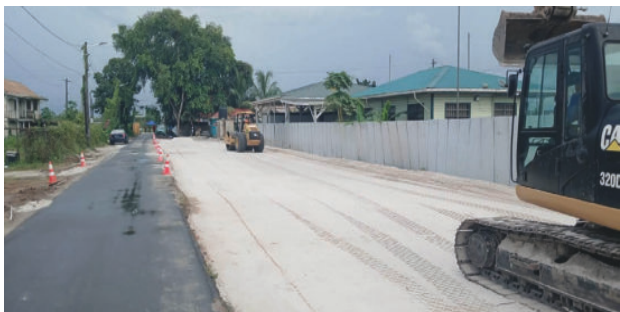
New Soesdyke Roundabout moves closer as preparatory works advance
