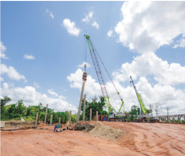
Permanent Puruni Bridge to strengthen Region 7’s productive economy
