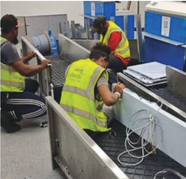
Works ongoing on the state-of-the-art baggage handling system at the Cheddi Jagan International Airport
