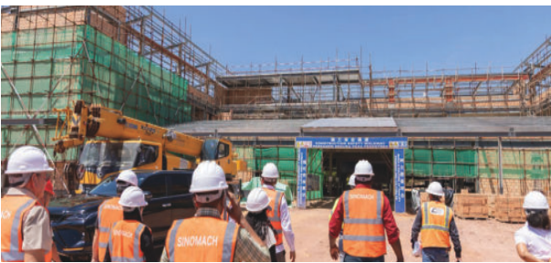
Construction ongoing on the new Lethem Regional Hospital
