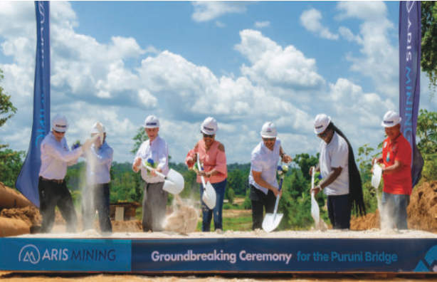
Permanent Puruni Bridge to strengthen Region 7’s productive economy
