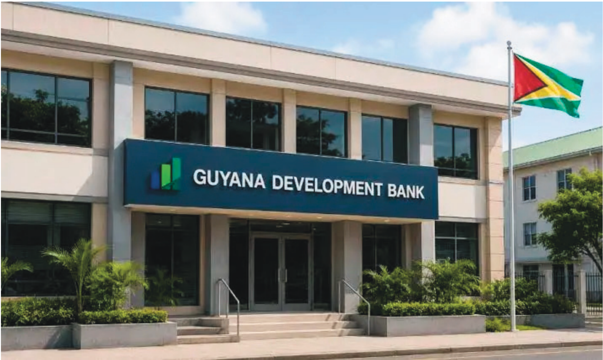
The Guyana Development Bank is now open for business
