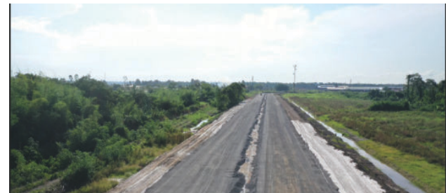
Craig-Land of Canaan highway advances, with 2027 completion targeted
