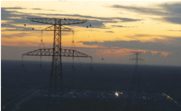
An electrical tower
