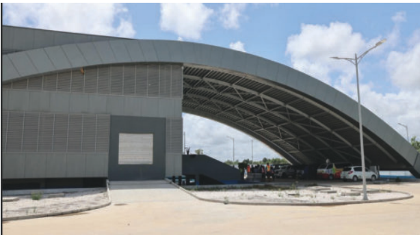
New US$20 million National Control Centre
