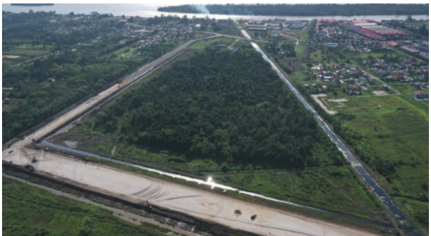
Craig-Land of Canaan highway advances, with 2027 completion targeted
