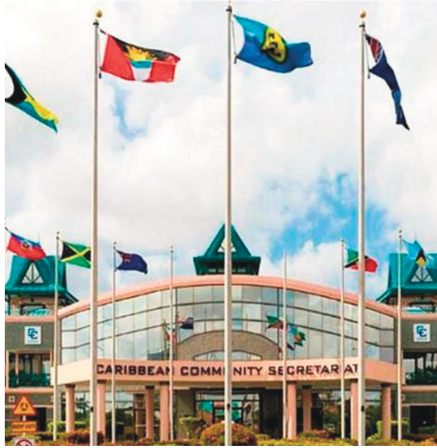
Caricom headquarters in Guyana
