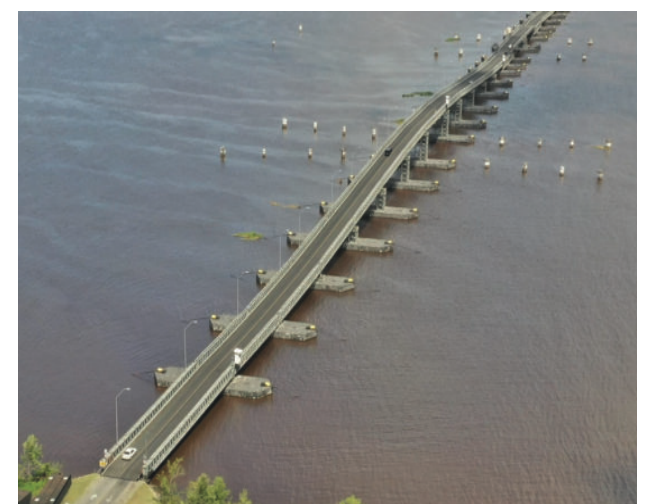
The Berbice River bridge
