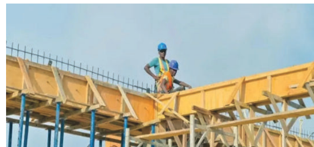
Construction is ongoing at the Tourism and Hospitality Institute in Port Mourant, Region Six
