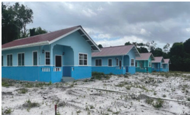
Some of the V-roof units at Block CHPA Development
