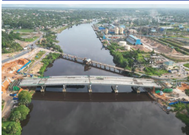
Aerial view of the progress on the construction
