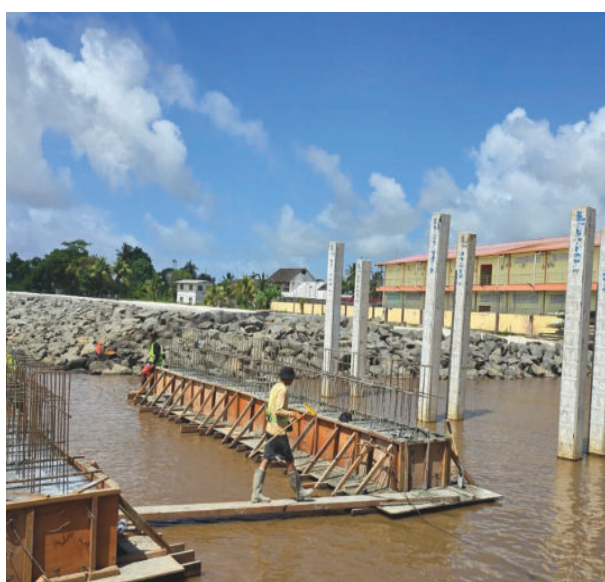
First concrete poured for Parika Port facility
