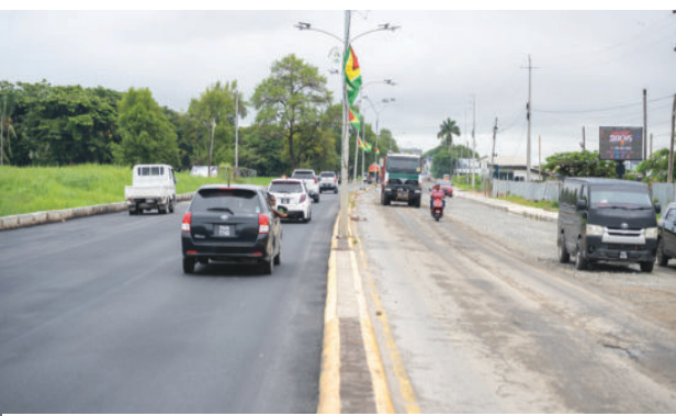
Carifesta Avenue Road Project progressing
