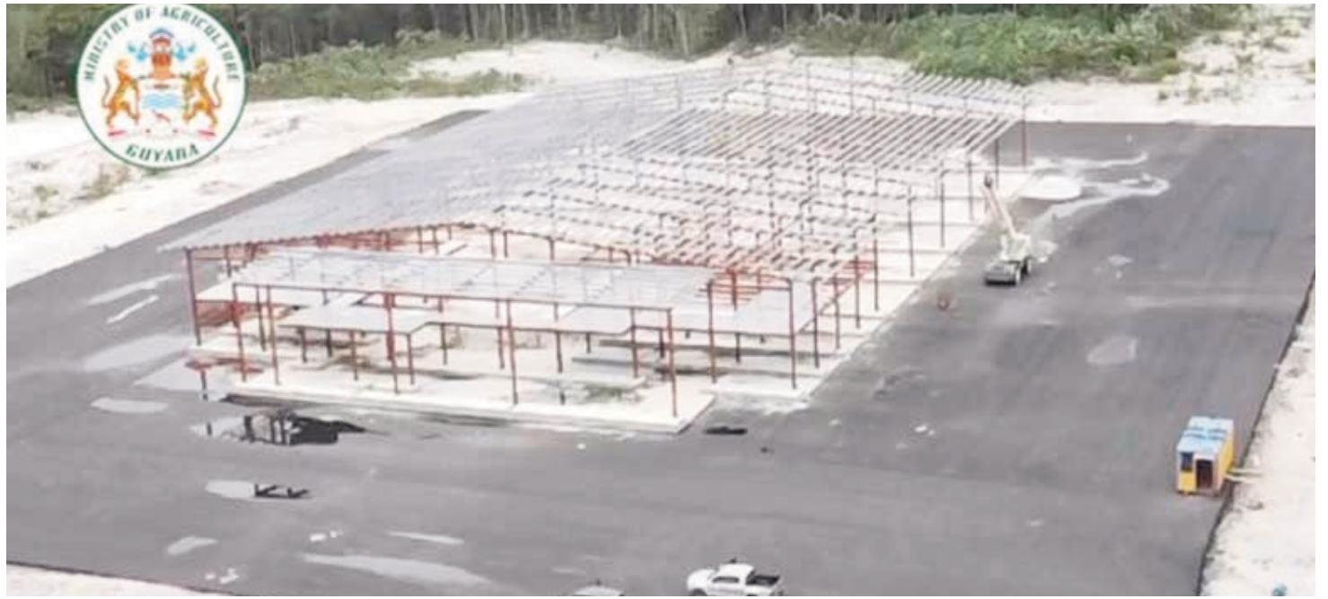
Construction continues at the Regional Food Hub at Yarrowkabra
