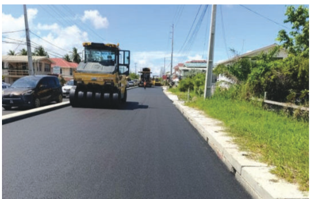
Ongoing construction on the East Coast Demerara road expansion project
