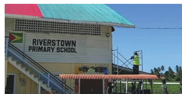
Repairs works conducted on affected homes and public buildings
