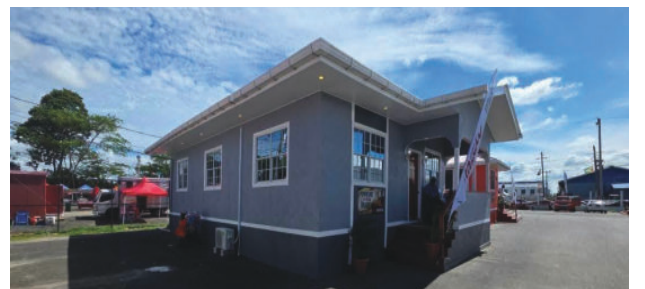
The Ministry of Housing - Central Housing and Planning Authority's model homes
