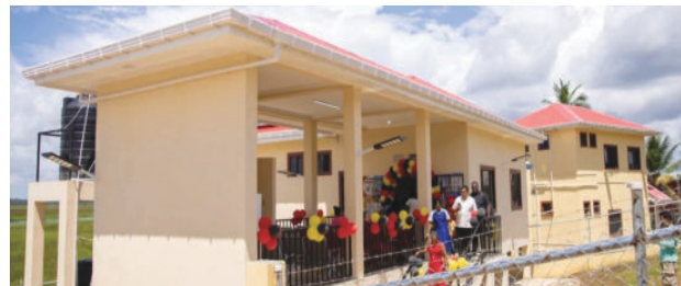
A new $30 million health centre and completed $30 million staff living quarters was commissioned at Red Hill.
