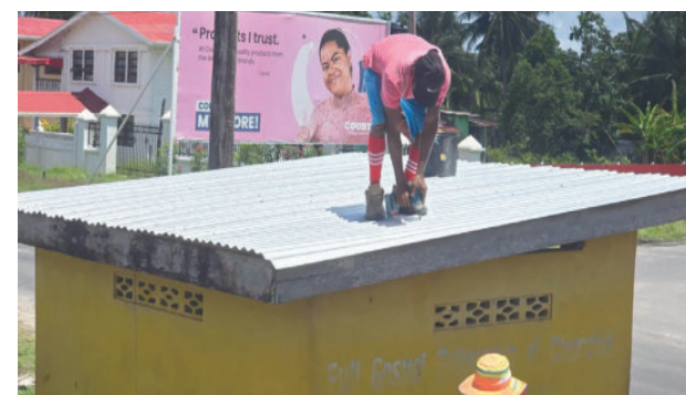
Repairs works conducted on affected homes and public buildings
