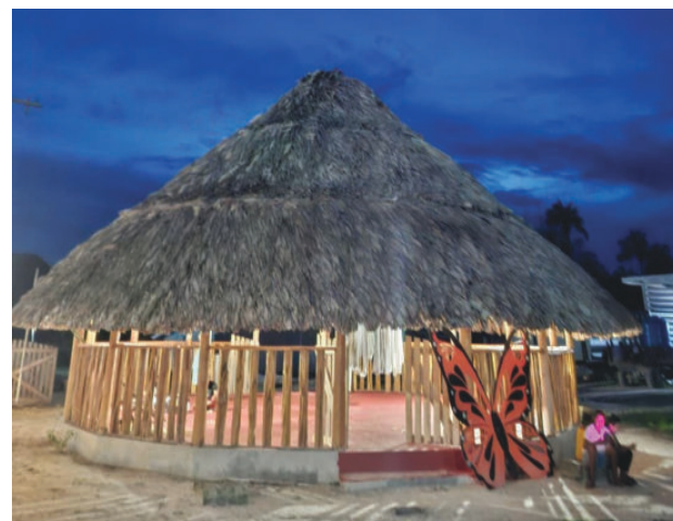
The newly constructed benab in St Deny
