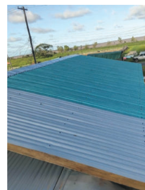
Repairs works conducted on affected homes and public buildings
