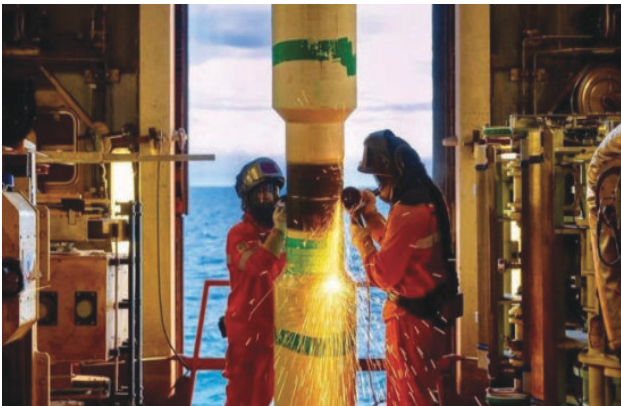
Welding onboard the Liza Destiny floating production storage and offloading (FPSO) – Guyana's first oil development
