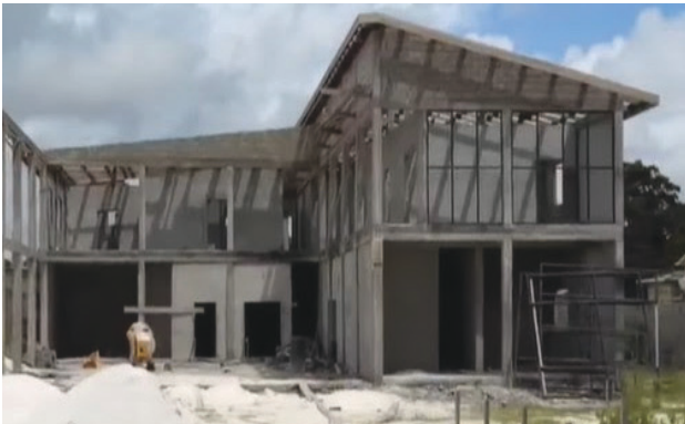
Onderneeming Fire Station under construction
