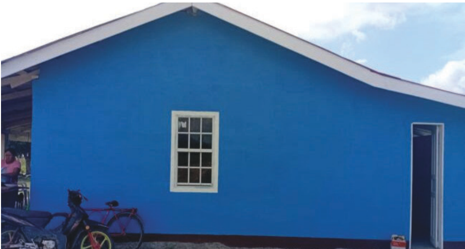
New $5M school kitchen at Bashaizon Village
