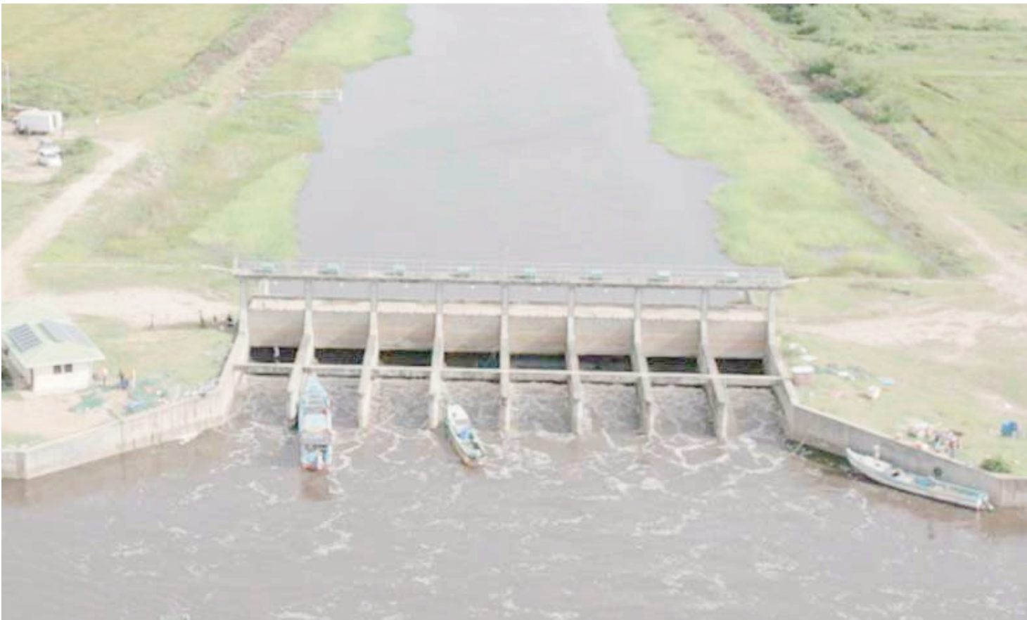
One of the flood control measures
