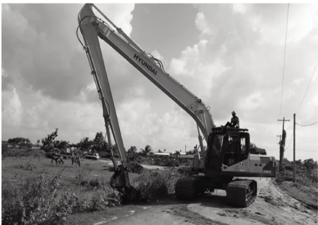
An excavator conducting drainage works
