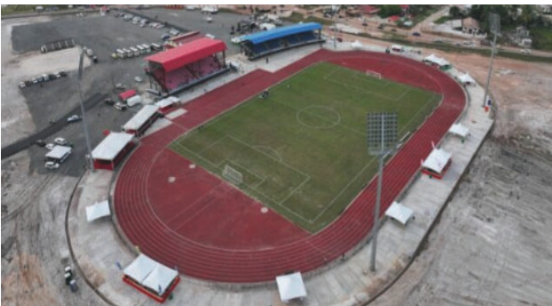
The Bayroc National Stadium.
