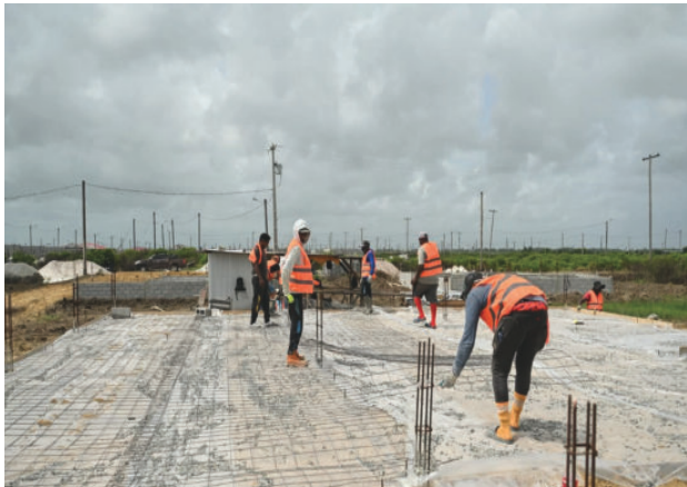
New roads, new communities taking shape as housing drive expands
