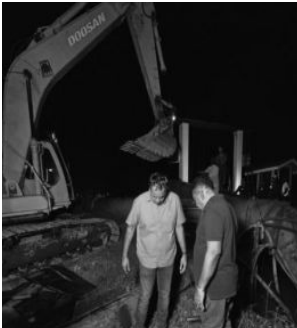
Schoonord’s flood defence restored after fishing boat collision
