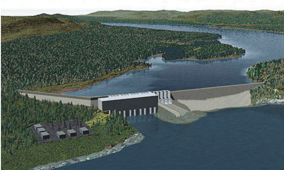
Churchill Falls Generating Station
