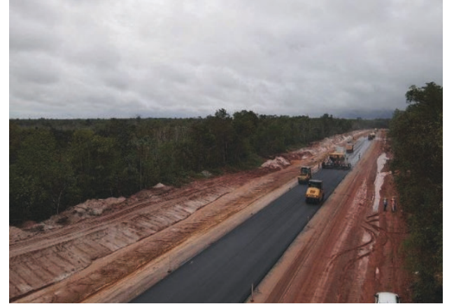
Drone shot of works on the road
