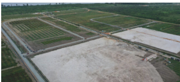
Drone image of Wales Commercial Zone under development
