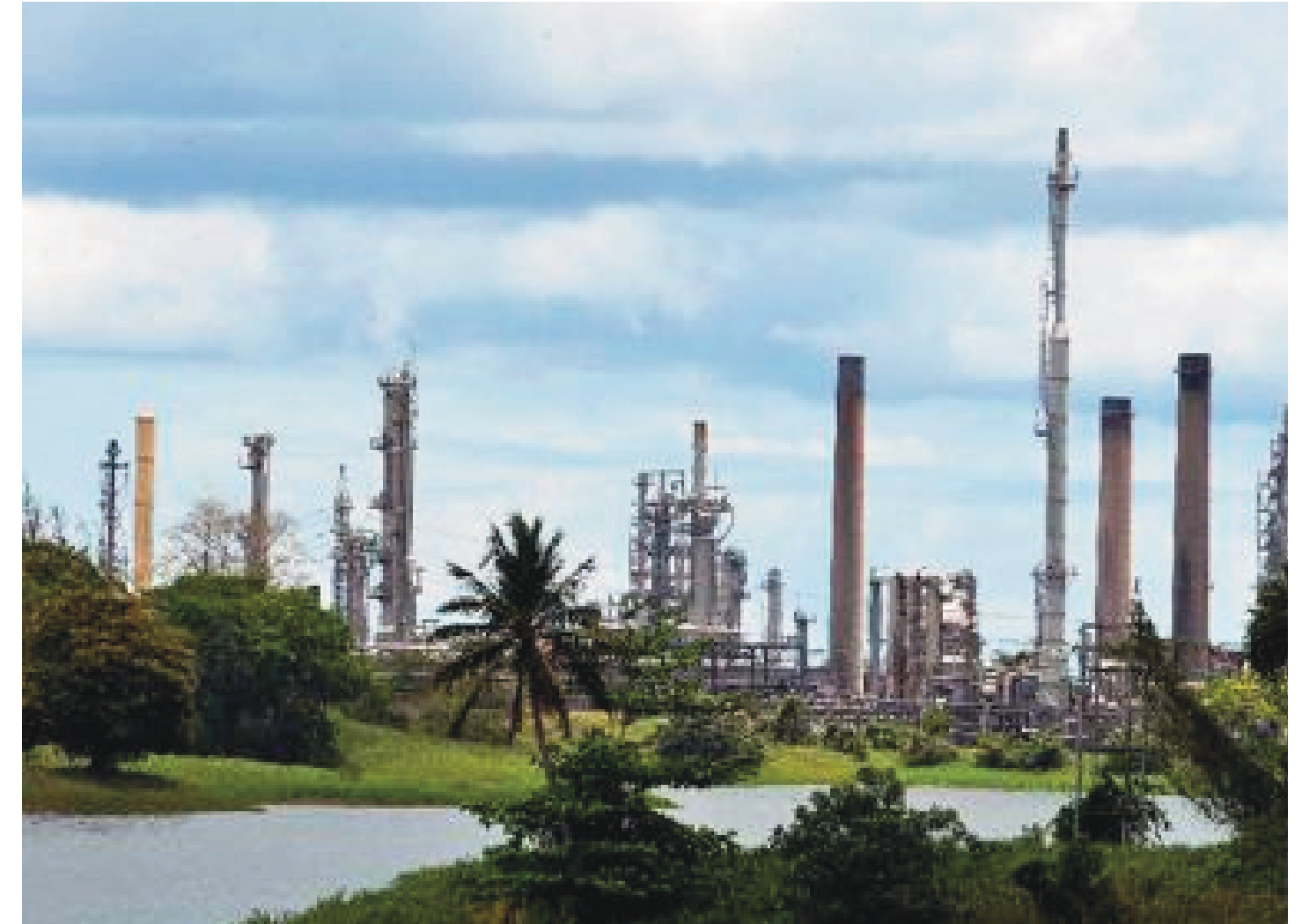
The Point-a-Pierre Refinery in Trinidad — in the process of being restored
