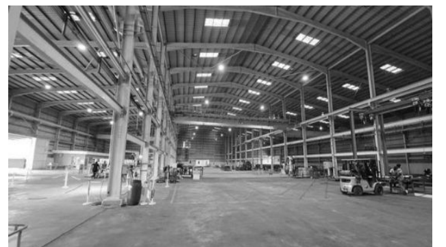
A tour of the Guysons K+B joint venture
