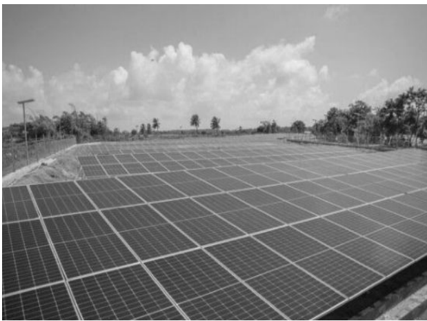
0.60 MW grid-forming solar photovoltaic farm in Leguan
