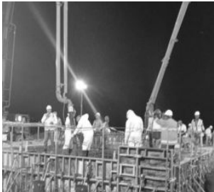
Pouring of the foundation for the first gas turbine at the transformative Gas-to-Energy facility in Wales, West Bank Demerara
