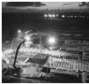
Pouring of the foundation for the first gas turbine at the transformative Gas-to-Energy facility in Wales, West Bank Demerara
