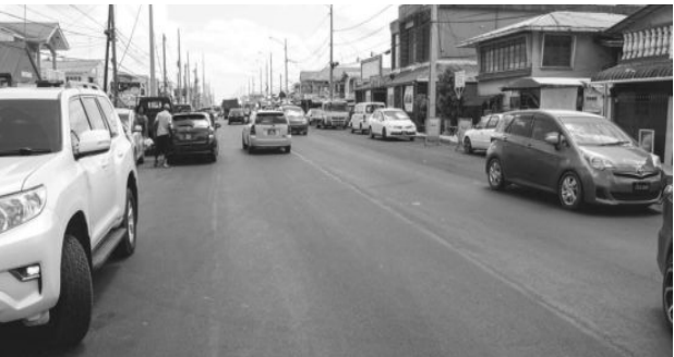
A section of the access road at Grove
