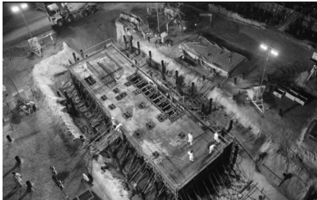
Another major concrete pour, recently took place at the site, marking steady progress on the project
