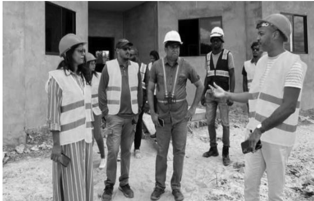
Construction progressing on the school
