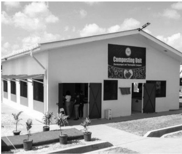
The newly commissioned Composting Unit at NAREI
