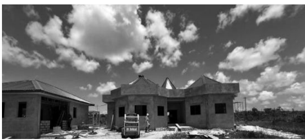
Construction progressing on the school
