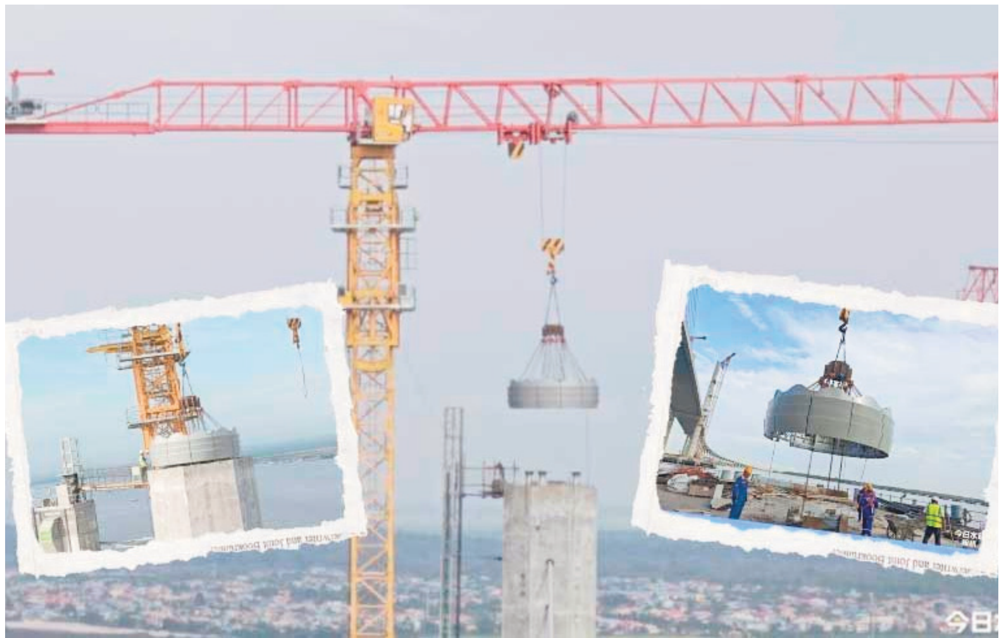
The crowns being installed on the iconic river bridge
