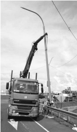
Street lights being installed on Sheriff Street
