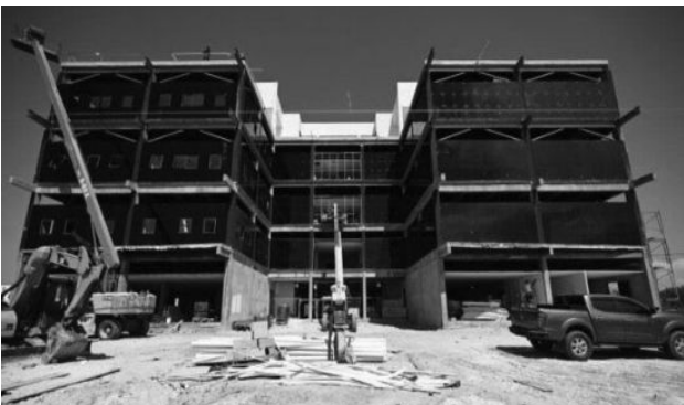
Construction on the new Headquarters of the Ministry of Housing progressing
