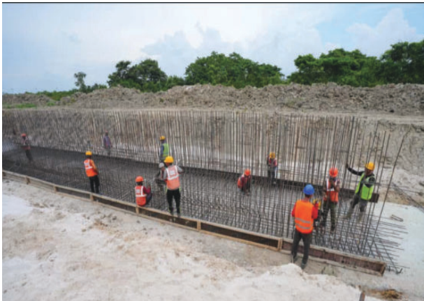
Scene from the inspection of the road projects
