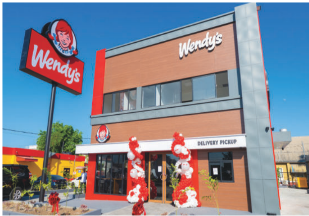
The flagship restaurant is located at the former KFC building on Vlissengen Road
