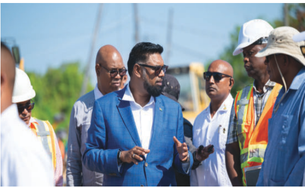
President Ali inspecting ongoing works on the East Coast road improvement project
