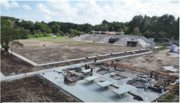
Construction work ongoing on the park
