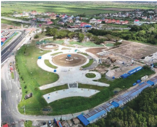
Construction work ongoing on the park
