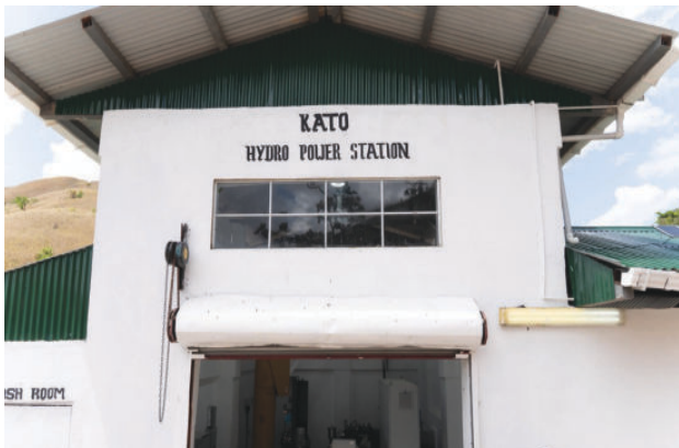
A new 0.15 MW hydropower plant has been commissioned in the village
