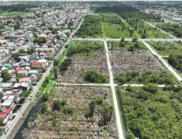
An aerial view of the ongoing works at the Le Repentir Cemetery
