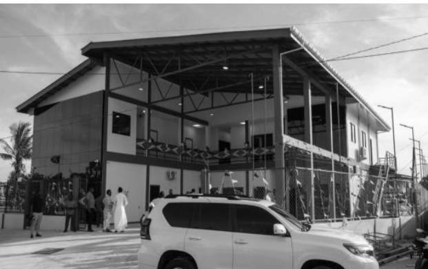
Parika welcomes state-of-the-art fire station
