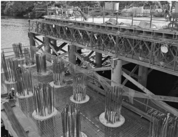
Ongoing work on the bridge
