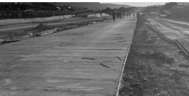
Ongoing works on the Paramakatoi airstrip
