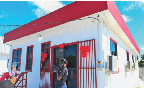
The facility aims to enhance service delivery and better meet the housing needs of residents in Regions Five and Six
