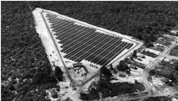
The commissioning of the 5MW Solar Farm at Onderneeming, Essequibo Coast
