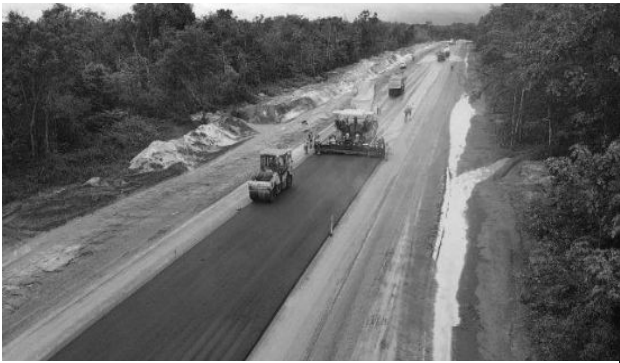
Drone shot of works on the Linden-Mabura road project
