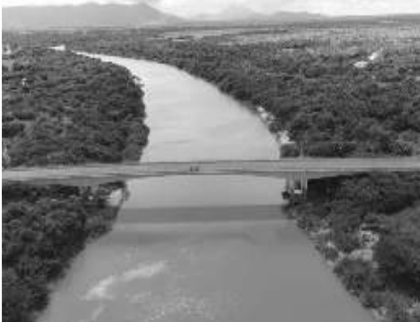
Completed in 2009, the Takutu River Bridge is a bridge across the Takutu River, linking Lethem in Guyana to Bonfim in Brazil
