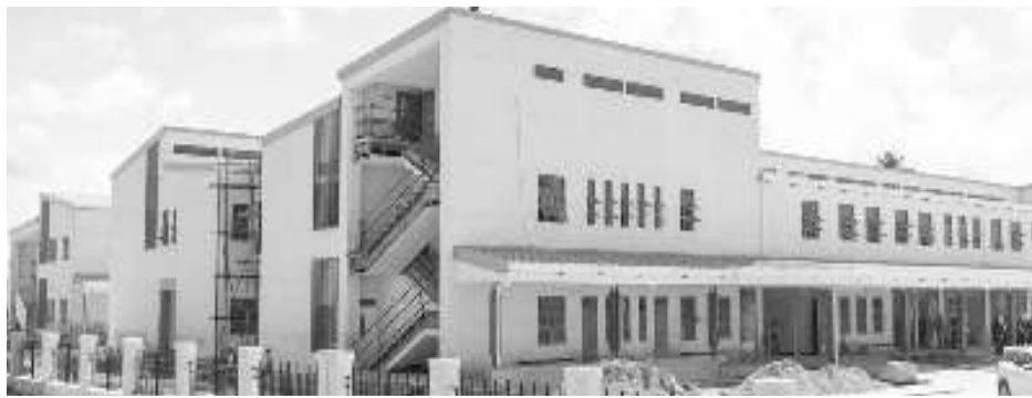
Scene from the Enmore Regional Hospital site visit
