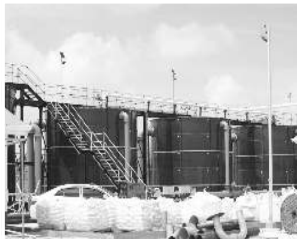
Onderneeming water treatment plant
