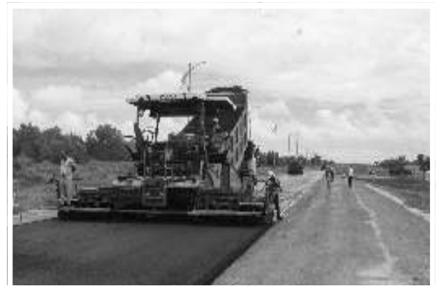
Paving works underway at the Ogle to Eccles bypass road project
