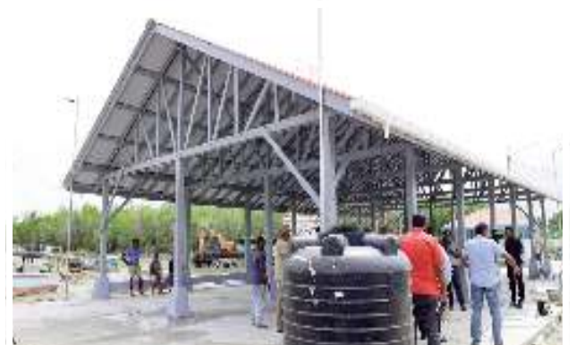
A section of the shed that was constructed
