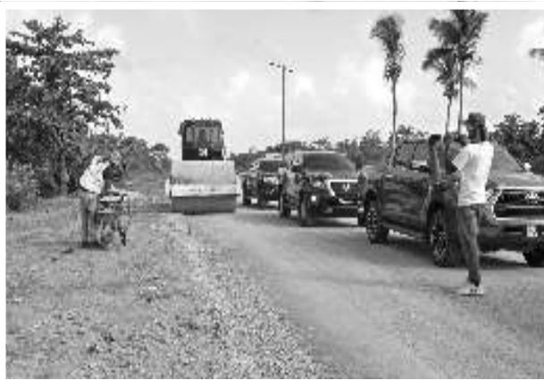
Ongoing works on the Mara road project
