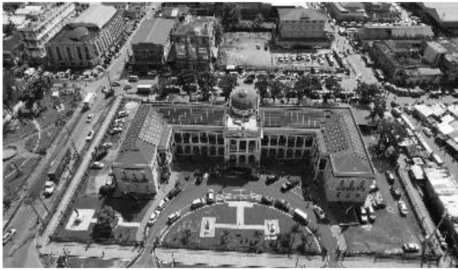
The project will retrofit approximately 500 public buildings across Guyana, Grenada, and Saint Lucia
