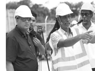
Minister of Housing and Water, Collin Croal, being provided with an update about Five Miles Water Treatment Plant
