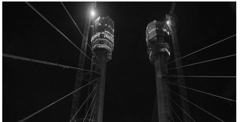
The final bridge tower (Pier 35) on the New Demerara River Bridge is completed
