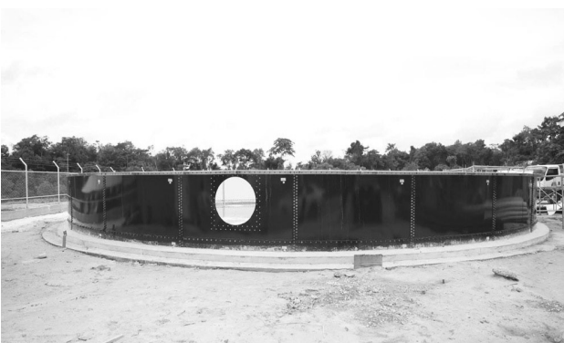
Five Miles water treatment plant
