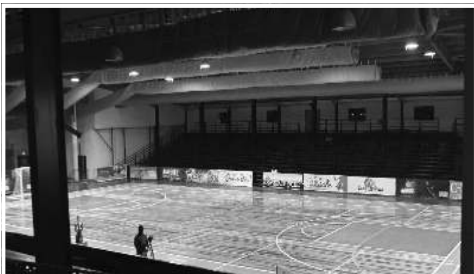
Work progressing on the Anna Regina Stadium in Region Two
