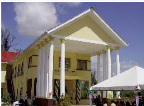
New state-of-the-art magistrates' court commissioned in Mahdia
