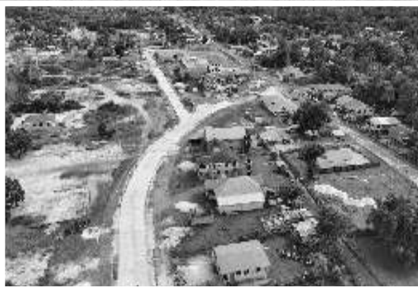
Ituni road upgrades
