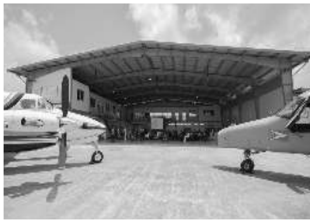
Part of the new facility
