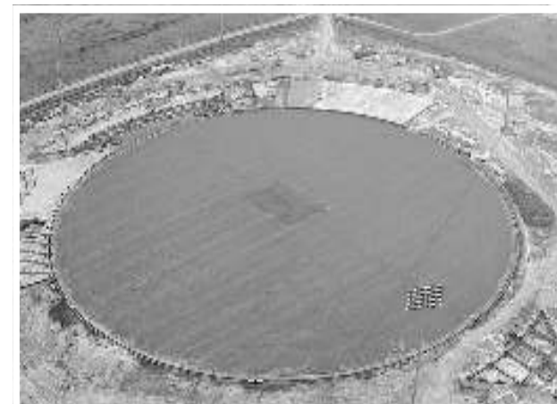
The stadium in Region Six taking shape
