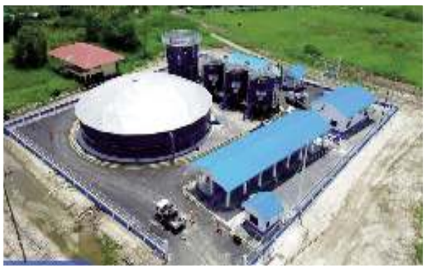
The massive $1.35 billion water treatment plant
