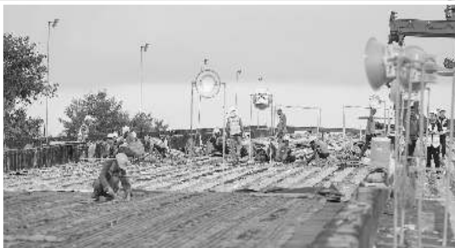
Some of the progress made on the bridge's construction
