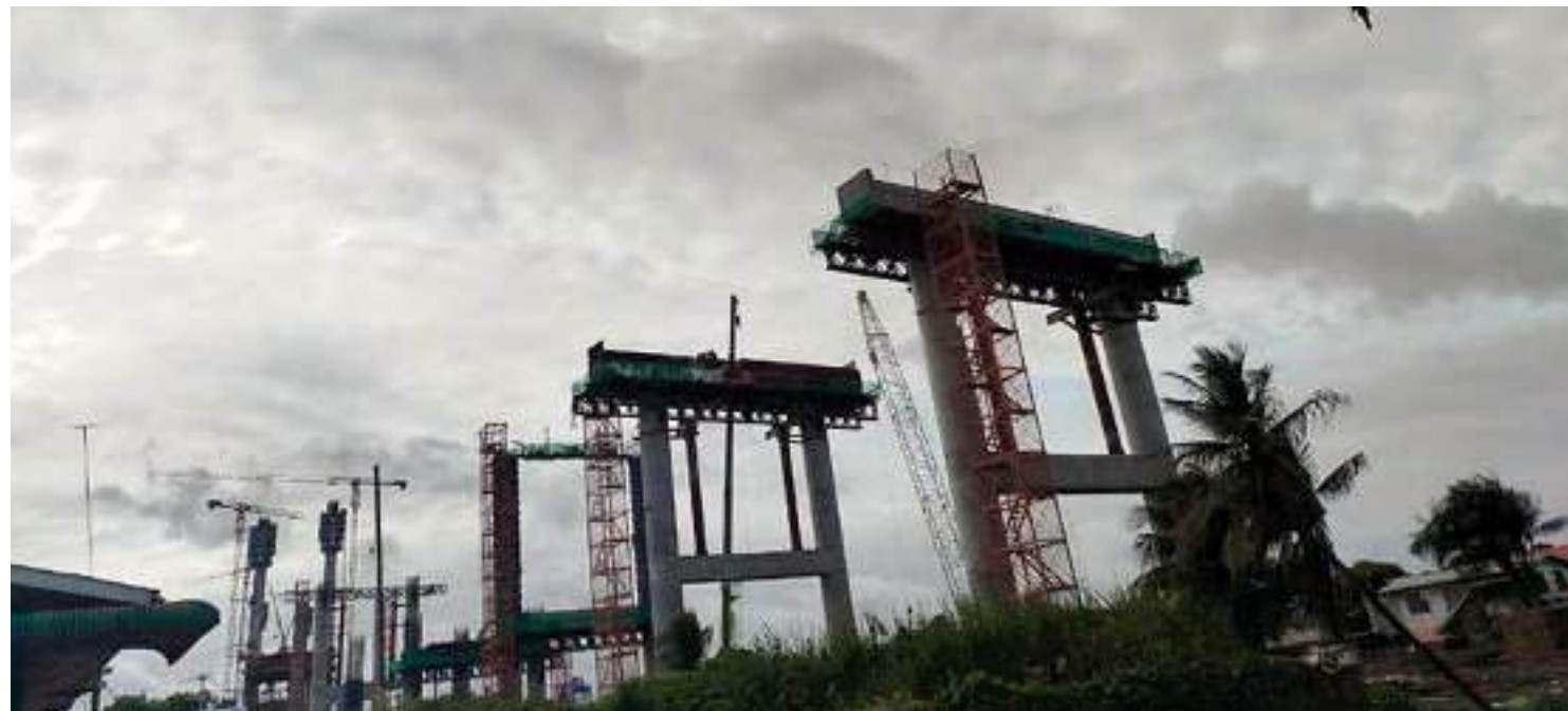
Ongoing work on the Demerara Harbour River Bridge
