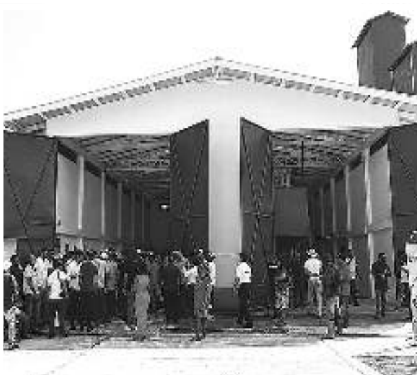
Scene from the commissioning of the seed processing facility
