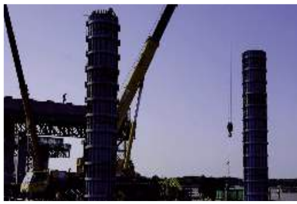
New Demerara harbour Bridge 64% completed
