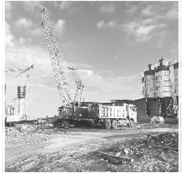
Ongoing works on the New Demerara Bridge
