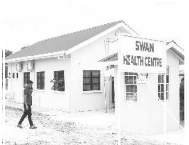
The new Swan Health Centre
