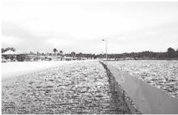
Creek operators are to implement immediate safety measures
