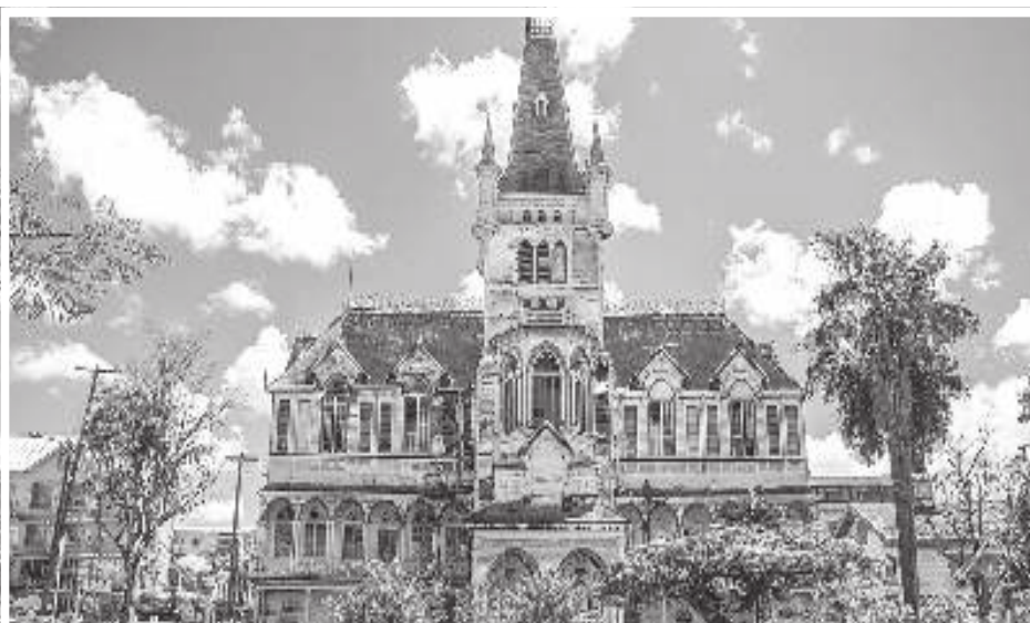
Georgetown City Hall has historically been the office of the mayor and city council
