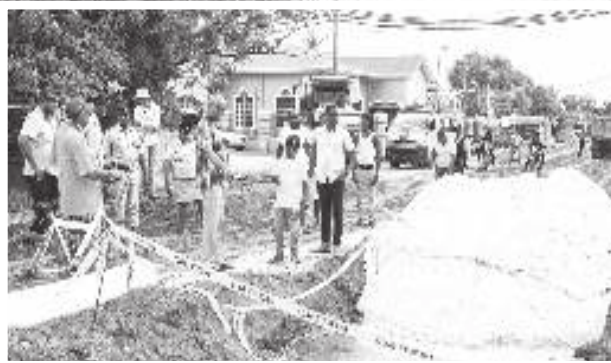
Ongoing restorative works on Lusignan road, East Coast Demerara
