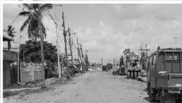
Ongoing works on the Conversation Tree Road Project
