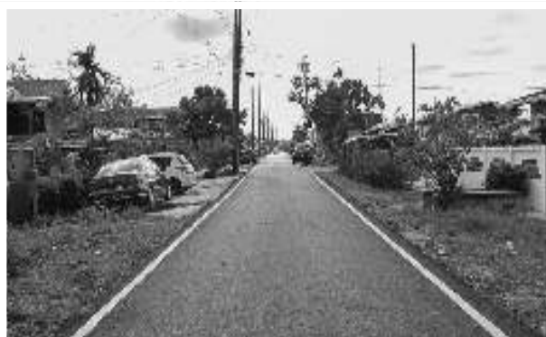
Road upgrade in Diamond, East Bank Demerara
