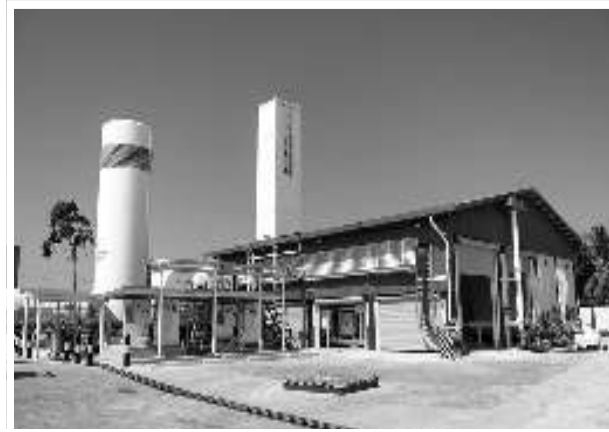
Massy Gas Products Guyana Ltd's Air Separation Unit
