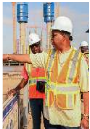
Minister of Public Works, Bishop Juan Edghill inspecting works at the eastern end of the new Demerara River Bridge
