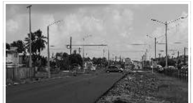
Ongoing works on the Conversation Tree Road Project
