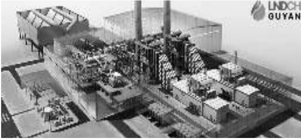
The Gas-to-Energy project will generate 2,100 gigawatt hours of electricity annual
