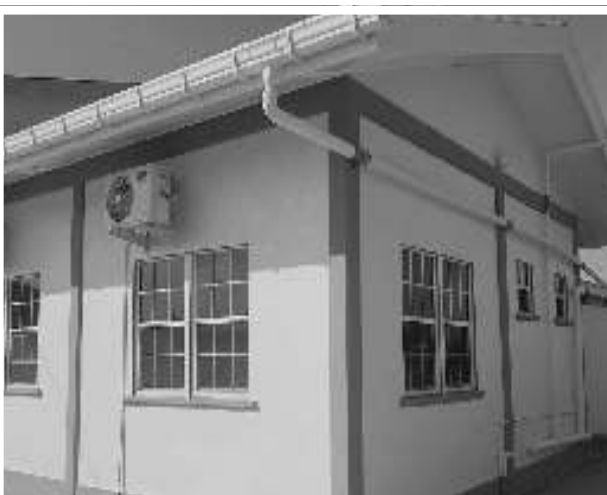
The newly expanded health facility
