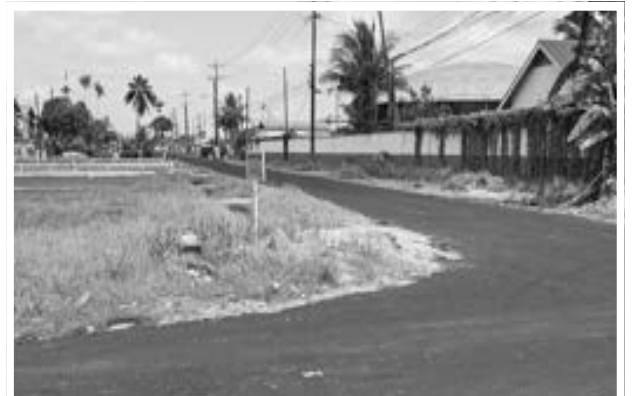
Road upgrade in Roxanne Burnham Gardens, Georgetown
