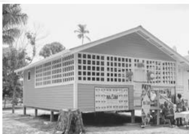
Santa Aratack, new community kitchen
