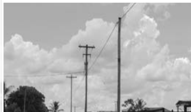
Some of the network lines that have been installed by GPL
