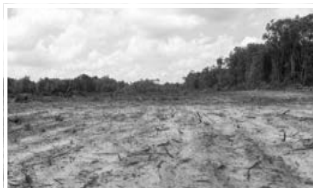
Infrastructure works underway at Hauraruni Housing Development
