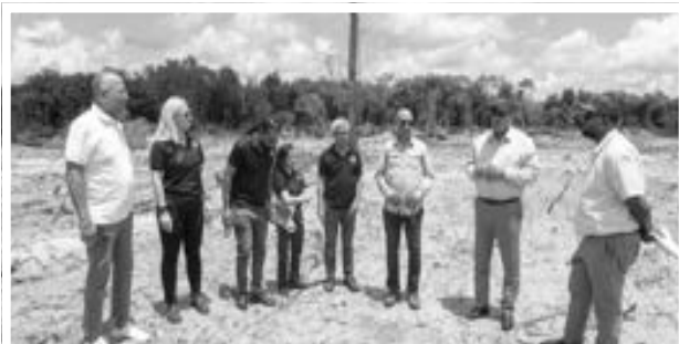
Land clearance ongoing to construct first 250 homes at Yarowkabra
