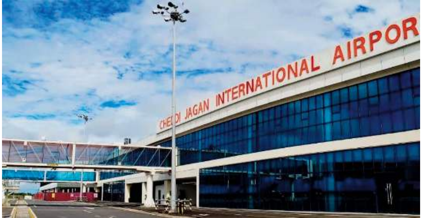
Over 1 million people will have arrived at the Cheddi Jagan Airport by November
