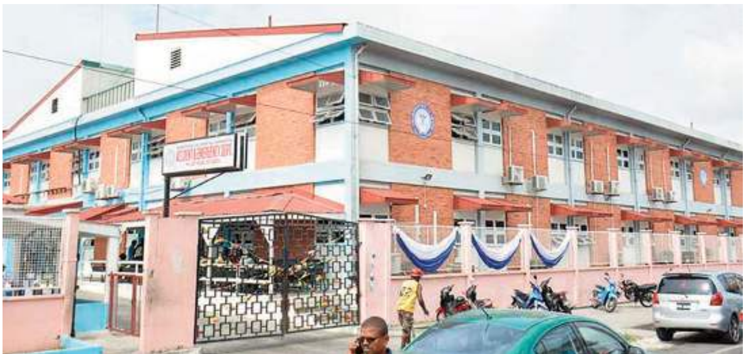
The Georgetown Public Hospital — getting major upgrades
