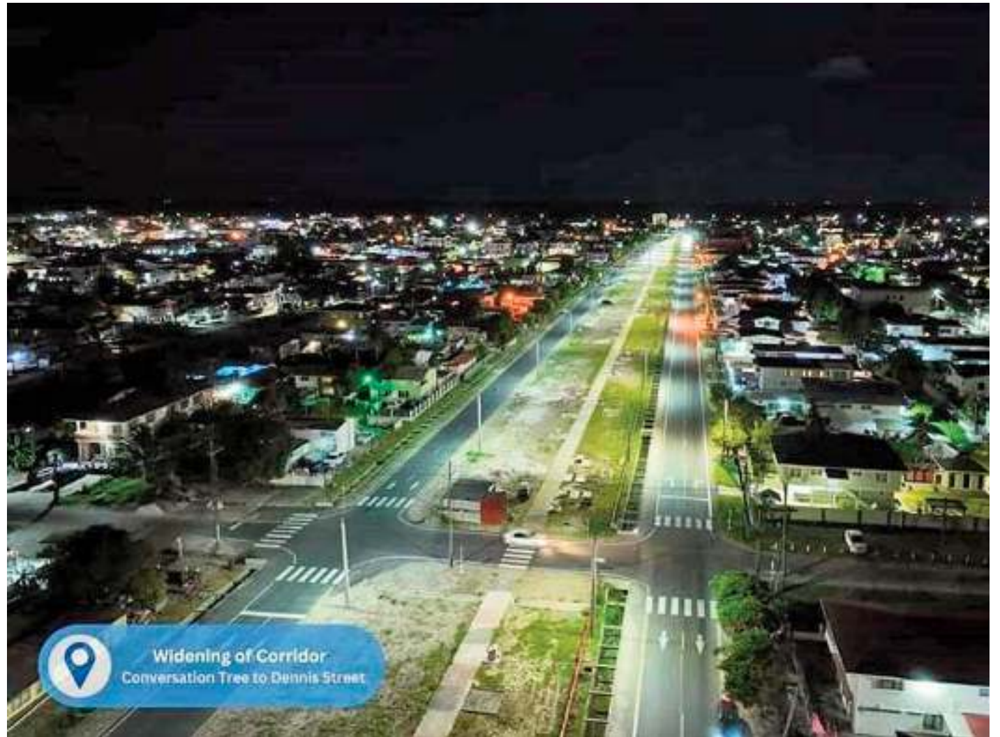
Aerial view of the newly constructed four-lane road from Conversation Tree to Dennis Street
