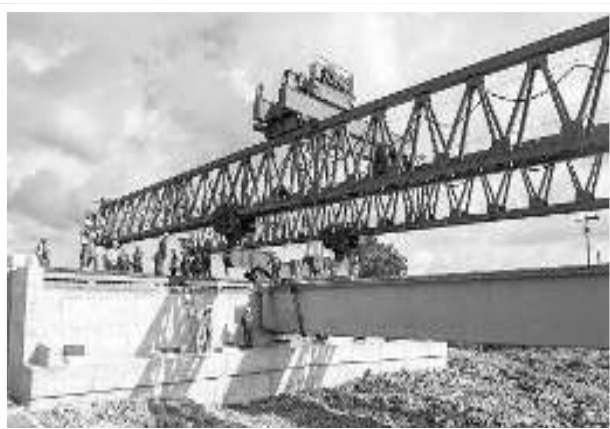
First precast girder installed for new Demerara River Bridge
