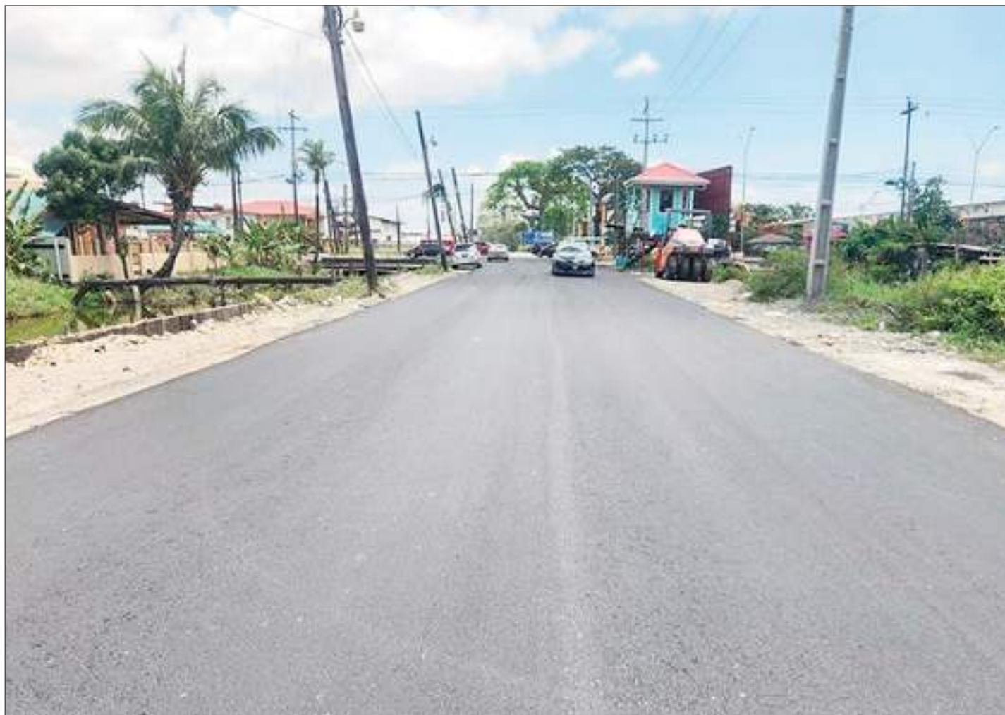
Rehabilitated Houston Industrial Zone Public Road
