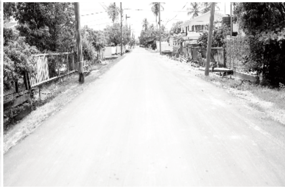
One of the newly constructed roads within Annandale village
