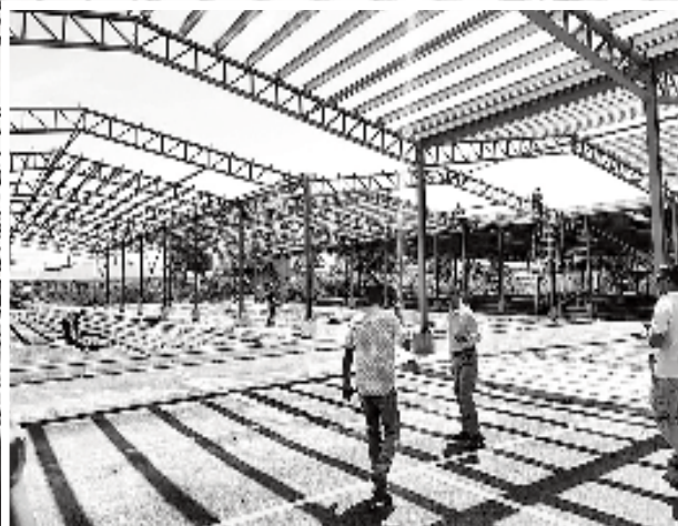
The Hydronie Market where works are nearing completion
