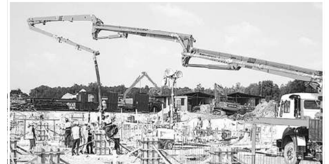
Construction of modern maternal and paediatric hospital progressing well
