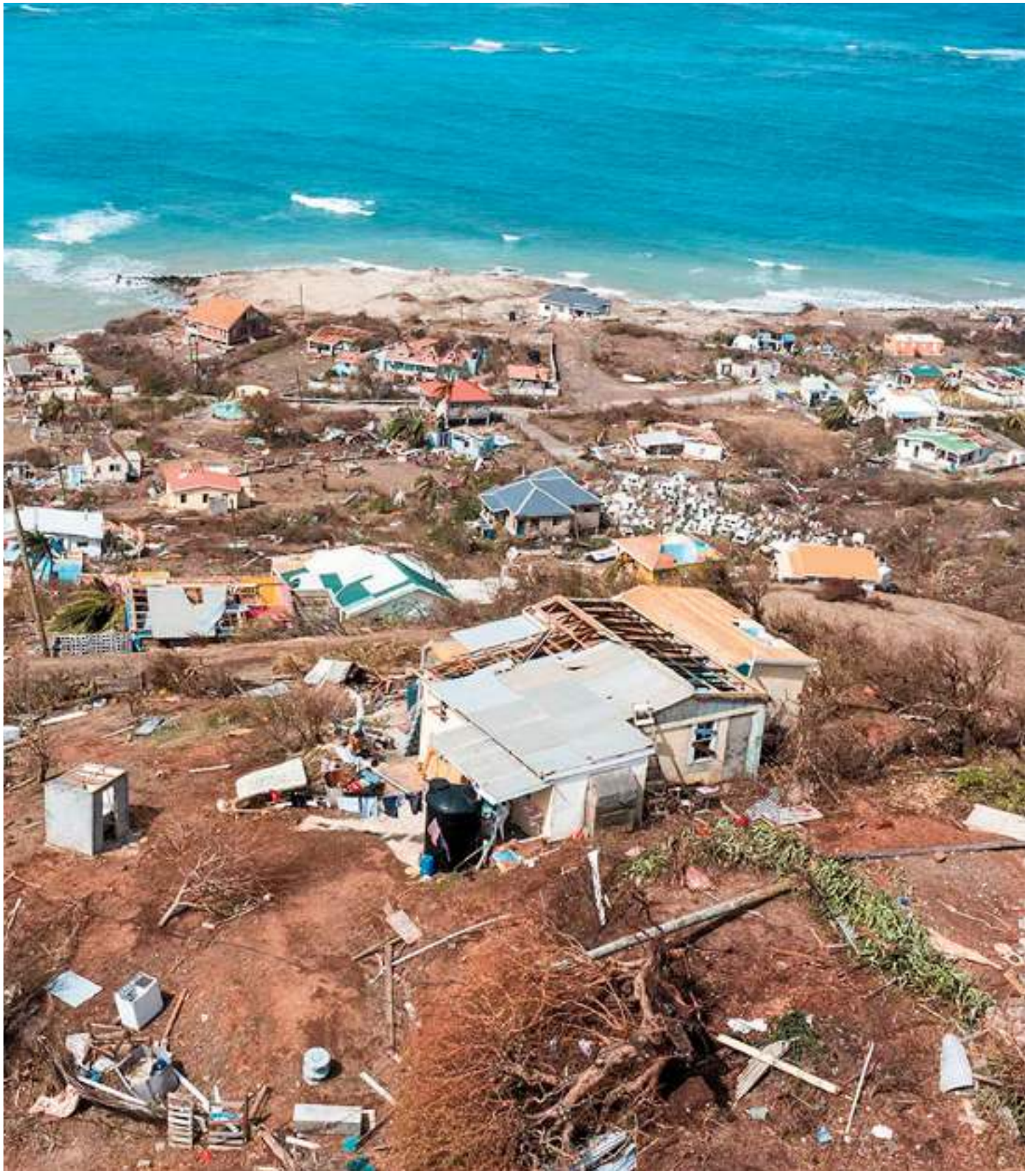
Damaged homes and buildings in Carriacou after Hurricane Beryl
