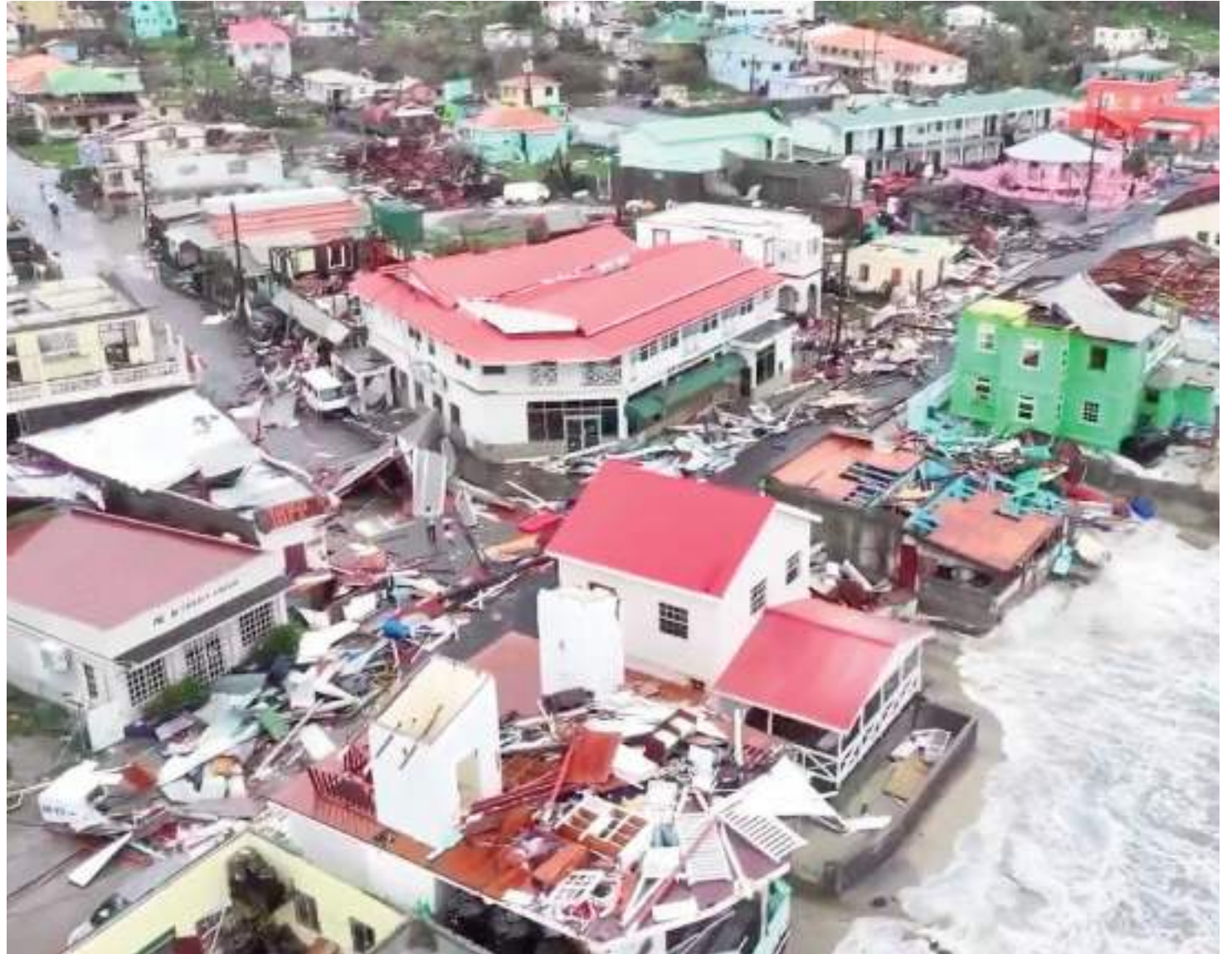
Damaged buildings in Grenada following the passage of Hurricane Beryl
