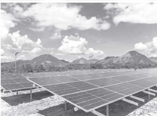
The Solar PV Mini-grid installed in Annai is a 41.5kW (ground-mounted) PV Array comprising 83 – 505Wp solar PV modules.
