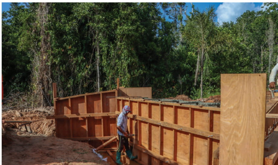
Works being done on Moblissa Bridge
