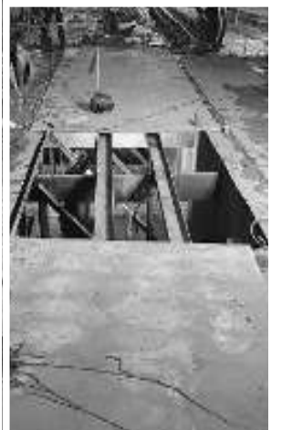
Workers carrying out repairs to the damaged barge back in June
