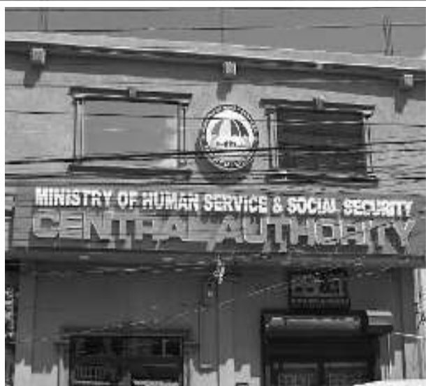
Guyana Central Authority building located in Albert Town
