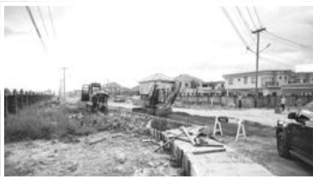
Massive infrastructural works taking place on the East Bank of Demerara
