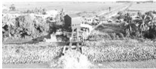
New $565.3M pump station commissioned at Greenwich Park, Region Three
