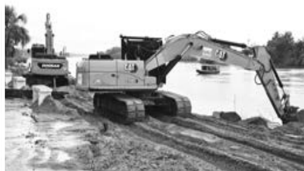
Ongoing River defence works on the Mackenzie watershore
