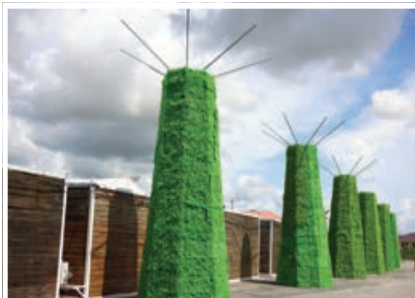
Ongoing works on the booths at the National Stadium
