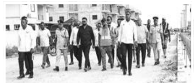
President Ali inspecting ongoing road works on the East Bank of Demerara
