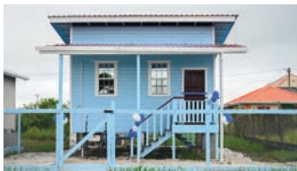
The newly constructed house that Hendricks will be moving into
