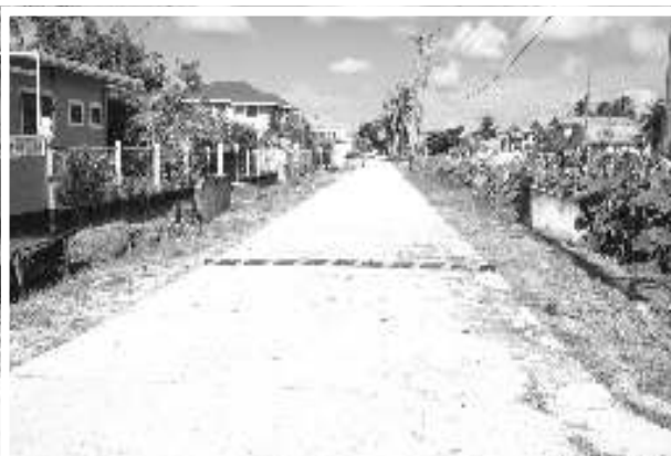
One of the completed roads
