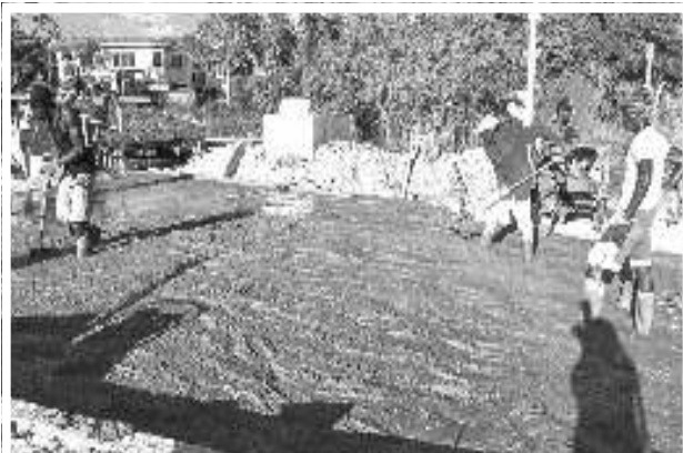
Works are ongoing on several roads
