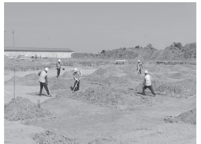
Workers levelling the ground for the new hospital
