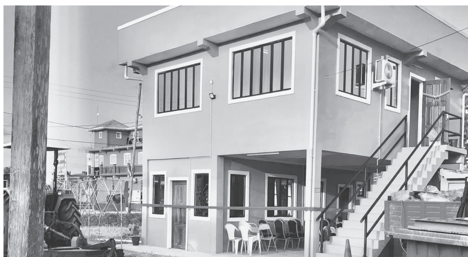
Newly commissioned Cane Grove NDC building
