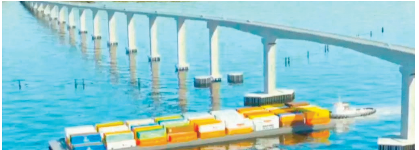
An artist impression of what the Corentyne River Bridge is expected to look like
