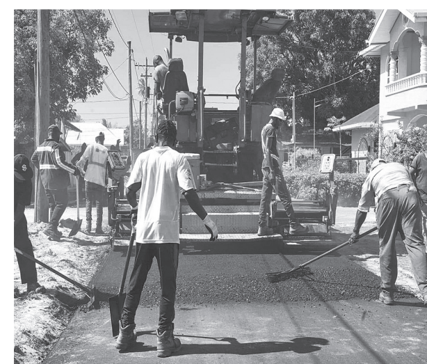
Road works in Enterprise, ECD
